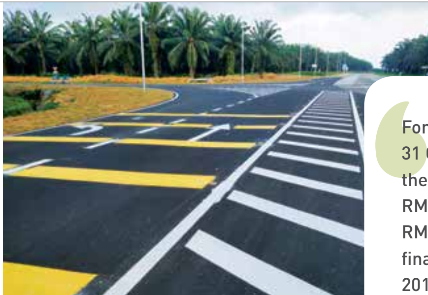
Completed access road to Cypark's SMART WTE plant
