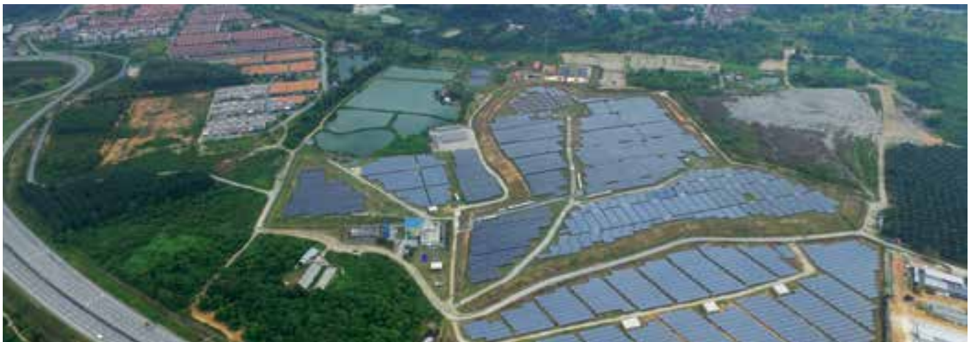
Cypark's Renewable Energy Park located in Pajam was developed and constructed under a remediated landfill area
