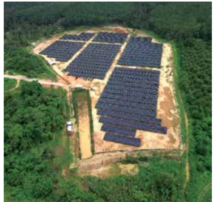
4.3 MWdc Renewable Energy Park in Jelebu, Negeri Sembilan
