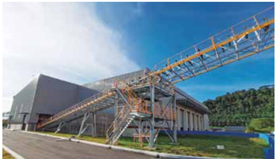
Waste Segregation Facility (WSF) in Ladang Tanah Merah, Negeri Sembilan
