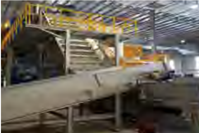
Waste Segregation Facility (WSF)
