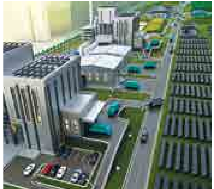
Waste-to-Energy Plant, Ladang Tanah Merah
