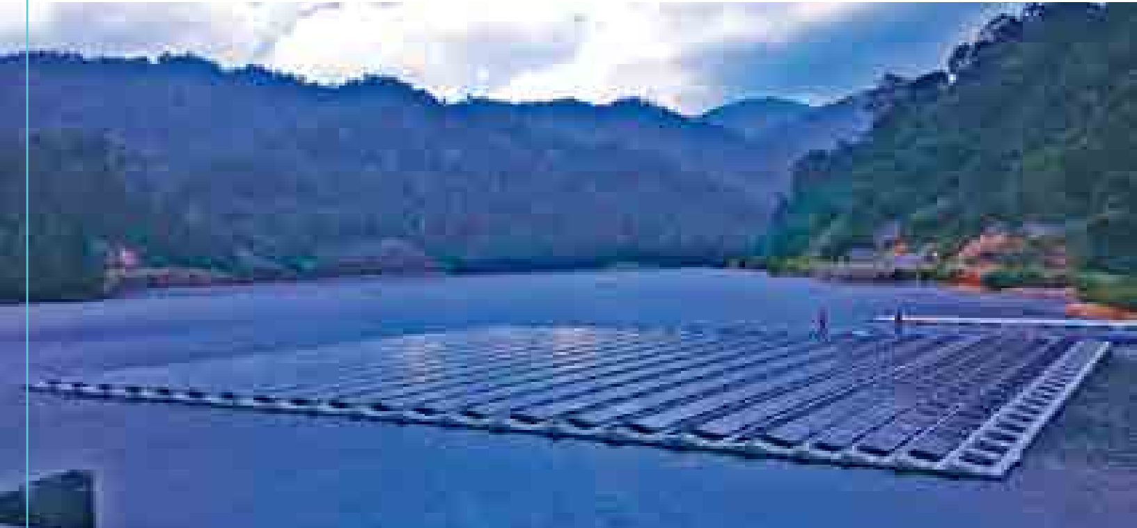
• Southeast Asia's Largest Floating Solar System at Empangan Sepri, Pedas, Negeri Sembilan
