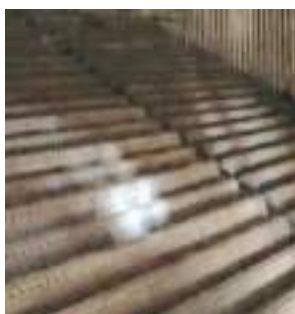
Moving Grate (Internal)
