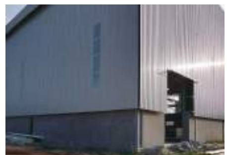
Waste Segregation Facility (WSF)
