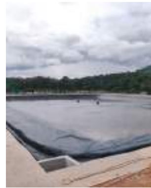
▶ Fully Anaerobic Bioreactor System (FABIOS) in Ladang Tanah Merah, Negeri Sembilan
