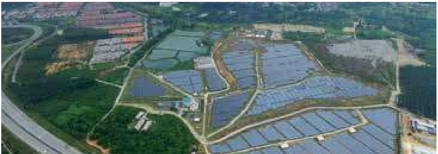
Cypark's Renewable Energy Park located in Pajam was developed and constructed under a remediated landfill area
