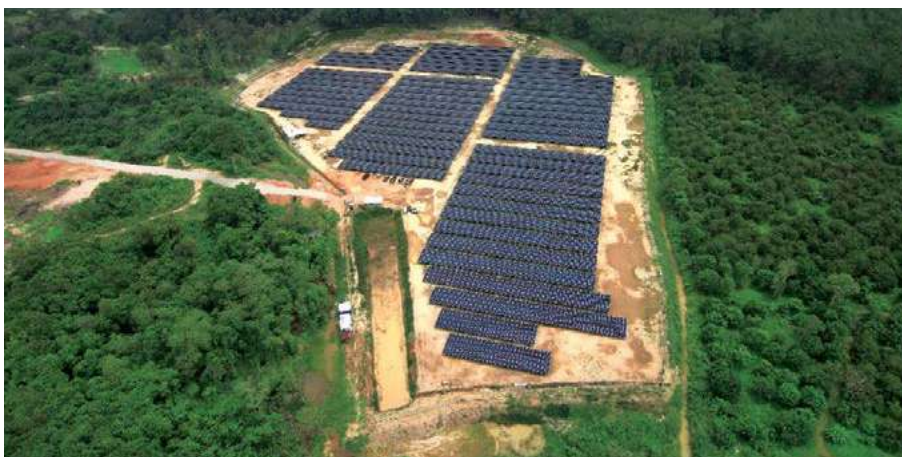
4.3 MW Renewable Energy Park in Jelevu, Negeri Sembilan
